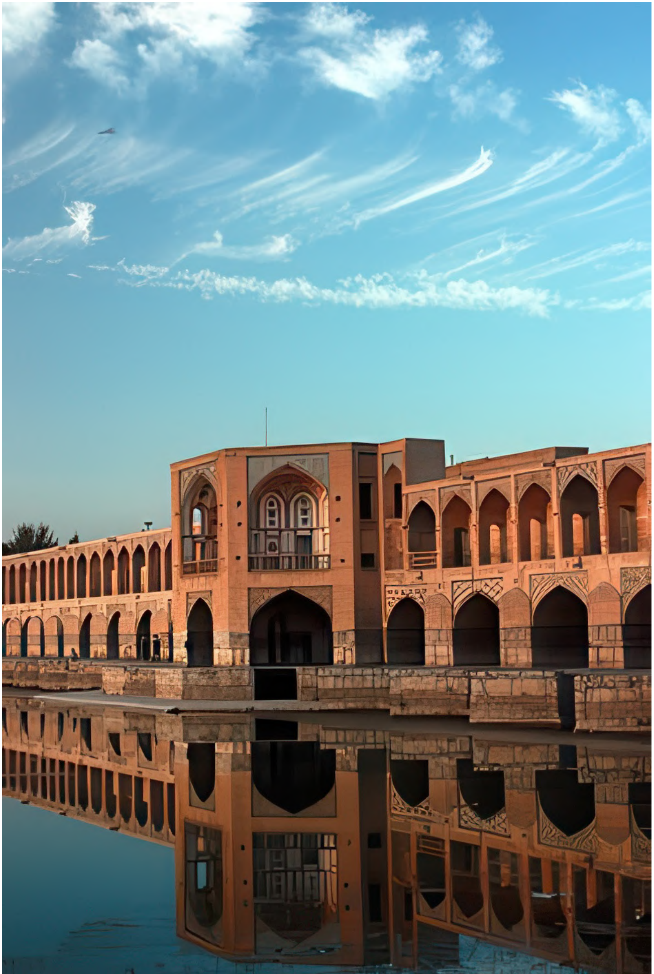
3. Khaju Bridge, Isfahan
